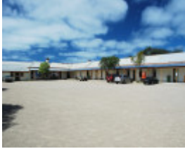
FORMER FORT FRANKLIN (PORTSEA CAMP) SOHE 2008
