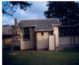
H02030 point nepean isolation hospital
