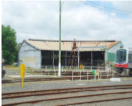
TRARALGON ENGINE SHED AND TURNTABLE SOHE 2008
