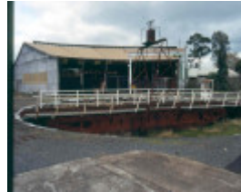
H01979 traralgon engine shed and turntable june 2001
