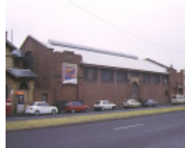
1 naval drill hall side view oct1997
