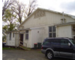
6168 Warragul Drill hall may07 ac 10
