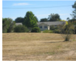
14247 Former Ballarat RAAF Base
