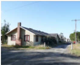
FORMER BALLARAT RAAF BASE SOHE 2008
