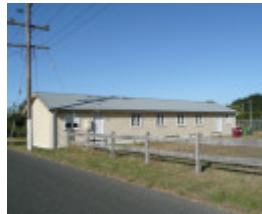
FORMER BALLARAT RAAF BASE SOHE 2008
