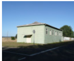
FORMER BALLARAT RAAF BASE SOHE 2008
