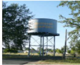
FORMER BALLARAT RAAF BASE SOHE 2008
