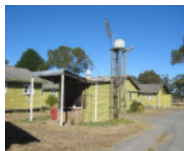
14247 Former Ballarat RAAF Base
