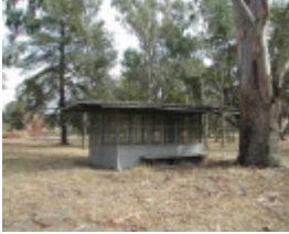
Shelter Shed, from the south east
