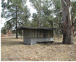
Shelter Shed, from the south east
