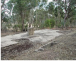
Concrete slabs, north west corner
