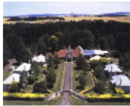
Rockbank Beam Wireless Station
