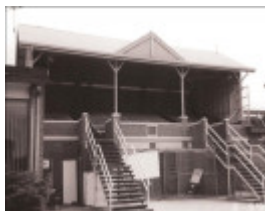
45617 Springvale Football Ground 01
