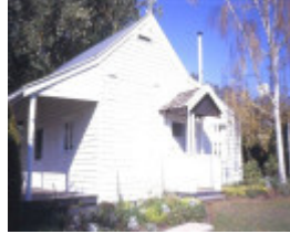
h00371 murrindindi station melba hwy yea canary cottage she project 2003
