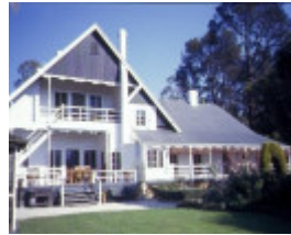
h00371 murrindindi station melba hwy yea homestead east elevation she project 2003
