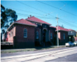
h02031 preston tramway workshops mess complex may03 aj
