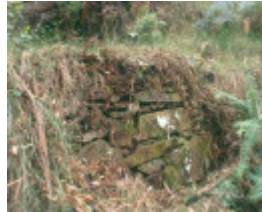
H02015 wheelers tramway retaining wall
