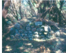
H02019 sealers cove saw mill stonework
