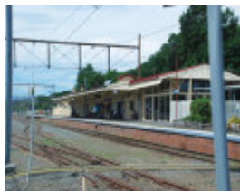
LILYDALE RAILWAY STATION REFRESHMENT ROOMS SOHE 2008
