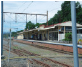
LILYDALE RAILWAY STATION REFRESHMENT ROOMS SOHE 2008
