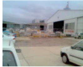
H0094 CAC hangars 2006
