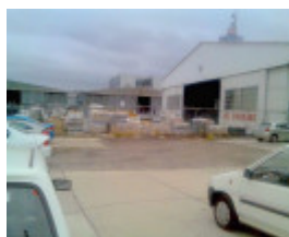
H0094 CAC hangars 2006
