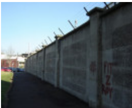
h00075 victoria park abbotsford june05 bath street concrete wall
