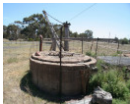
Brick vat Eucalyptus Factory Inglewood Oct 2006
