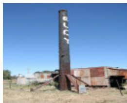
Chimney Eucalyptus Factory Inglewood Oct 2006
