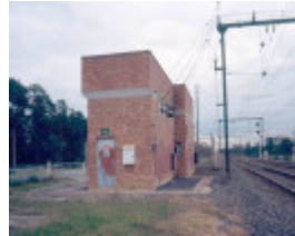
h02025 1 bunyip sub stationjul03 jc
