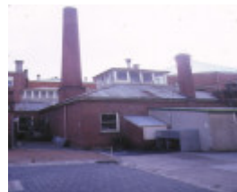
former sandhurst mechanics institute bendigo workshops aug1983
