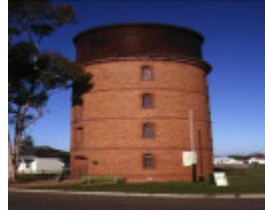
1 former railway water tower comyn avenue murtoa front view
