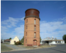
FORMER RAILWAY WATER TOWER SOHE 2008
