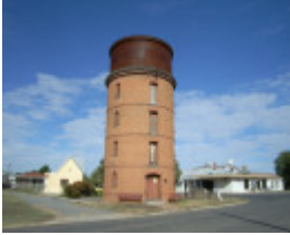
FORMER RAILWAY WATER TOWER SOHE 2008
