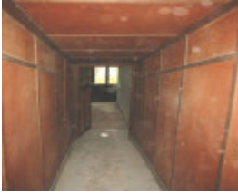
h01033 east view heidleberg tunnel nov2004 mz
