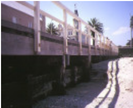
pier off kerford road albert park side detail
