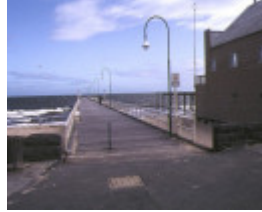
1 pier off kerford road albert park front view sep1992
