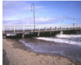
pier off kerford road albert park side view sep1992
