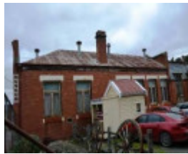
CMP Tech Addition north elevation (Source: CMP, 2021)
