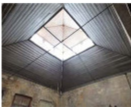
Room 10 ceiling detail (Source: CMP, 2021)
