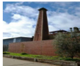
Laboratory building, assay chimney and roof light from west (Source: CMP, 2021)
