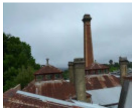
Laboratory building, assay chimney and roof lights from east
