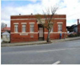
Vincent Street facade (Technical School Addition) (Source: CMP, 2021)
