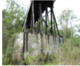
Murrindal truss bridge on cutwater IMG_0939.jpg
