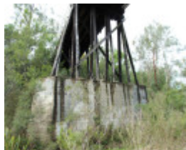
Murrindal truss bridge on cutwater IMG_0939.jpg
