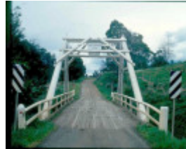
h02069 hiawatha bridge 1
