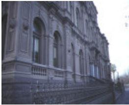
law courts bendigo facade detail jul1984
