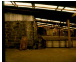
Sunnyside Wool Scour Interior
