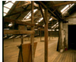
Sunnyside Wool Scour Interior
