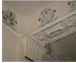
Ground Floor Hall, detail of decoration 2011
