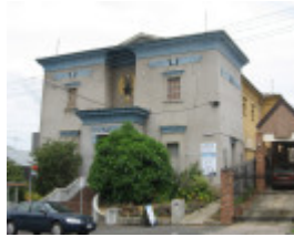
General view from north east 2011
