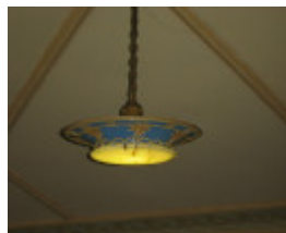
Lodge Room, light fitting 2011
