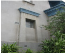
detail of window, front facade 2011
