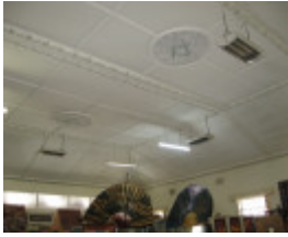
First floor foyer ceiling 2011
