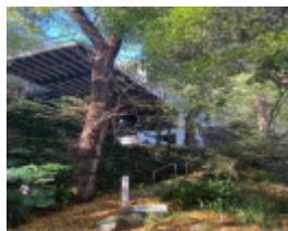
2023 cantilevering western end of River House
