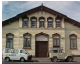
H01949 ranger barracks ballarat rear pm1 jan00 2
