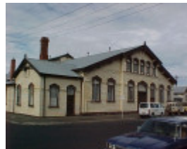
H01949 ranger barracks ballarat rear pm1 jan00
