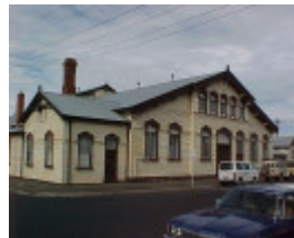
H01949 ranger barracks ballarat rear pm1 jan00
