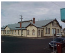
H01949 ranger barracks ballarat rear pm1 jan00 3
