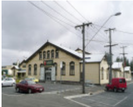
RANGER BARRACKS SOHE 2008
