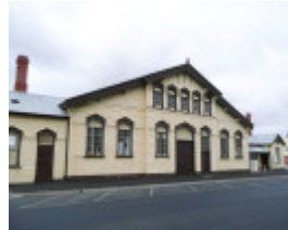
RANGER BARRACKS SOHE 2008
