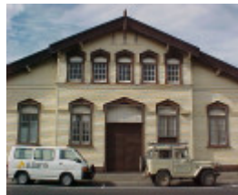
H01949 ranger barracks ballarat rear pm1 jan00 2
