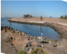
Power Station Park Seawall Williamstown March 2003
