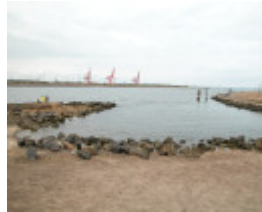
Yarra River Entrance Training Wall Williamstown March 2003 003
