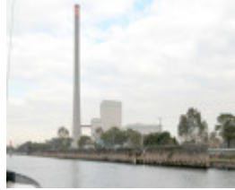
Newport Coal Wharves Williamstown Aug 2003 003
