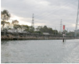
Newport Coal Wharves Williamstown Aug 2003 001
