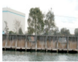
Newport Coal Wharves Williamstown Aug 2003 002
