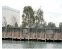
Newport Coal Wharves Williamstown Aug 2003 002
