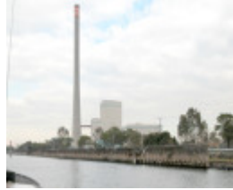
Newport Coal Wharves Williamstown Aug 2003 003
