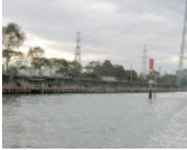
Newport Coal Wharves Williamstown Aug 2003 001
