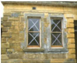
former supreme court now bendigo secondary college bendigo window detail sep1993
