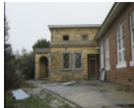
former supreme court now bendigo secondary college bendigo side view sep1993
