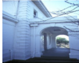
1 former supreme court now bendigo secondary college bendigo side entrance jul1984
