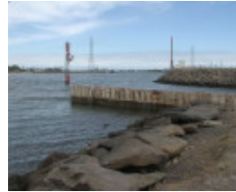
Channel Deepening Project
