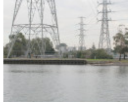
Newport Oil Wharves Williamstown June 2003 003
