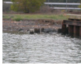
Newport Oil Wharves Williamstown June 2003 002
