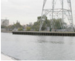
Newport Oil Wharves Williamstown June 2003 001
