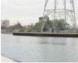
Newport Oil Wharves Williamstown June 2003 001
