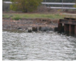
Newport Oil Wharves Williamstown June 2003 002
