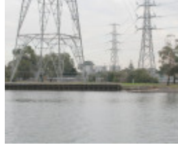
Newport Oil Wharves Williamstown June 2003 003
