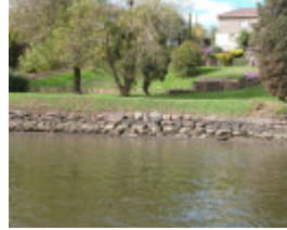
Jone's Slipway And Boatbuilding Yard Maribyrnong May 2003 002
