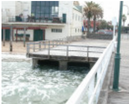
Kerferd Road Pier Port Melbourne March 2003 drain 004
