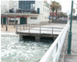
Kerferd Road Pier Port Melbourne March 2003 drain 004
