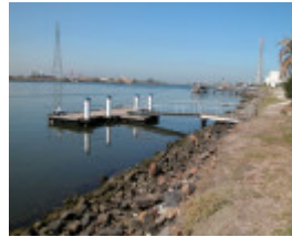
Spotswood Pumping Station Wharf Piles Williamstown May 2003 BoatLanding
