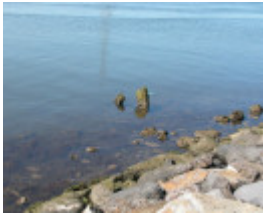
Spotswood Pumping Station Wharf Piles Williamstown May 2003
