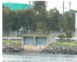
Spotswood Pumping Station Wharf Piles Williamstown May 2003 Overflow Outlet 002
