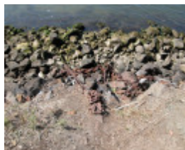
Spotswood Pumping Station Wharf Piles Williamstown May 2003 Mooring Cables
