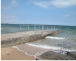
McGregor Street Drain Culvert Port Melbourne March 2003
