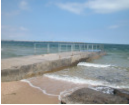
McGregor Street Drain Culvert Port Melbourne March 2003
