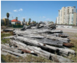
Princes Pier Port Melbourne March 2003 004
