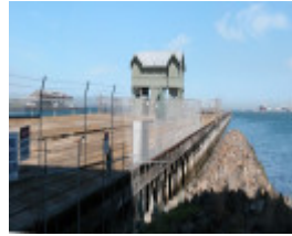
Princes Pier Port Melbourne March 2003 003
