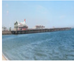
Princes Pier Port Melbourne March 2003 001
