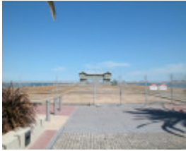
Princes Pier Port Melbourne March 2003 002
