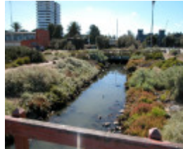
Cowderoy Street Drain Culvert Williamstown April 2003 view East 003
