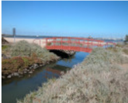
Cowderoy Street Drain Culvert Williamstown April 2003 Bridge Crossing 001
