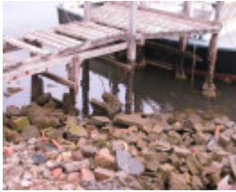
Koroit Creek Fishers Retreat Williamstown March 2003 closeup
