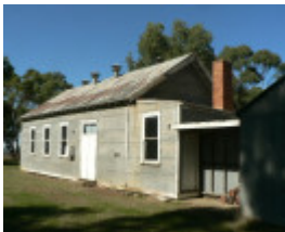
Gringegalgon Soldiers Memorial Hall - viewed from north-west
