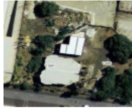
Maribyrnong substation aerial view
