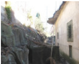
Maribyrnong substation quarry wall at rear
