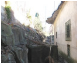
Maribyrnong substation quarry wall at rear
