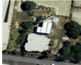
Maribyrnong substation aerial view
