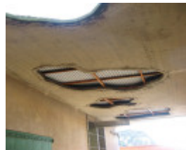
Maribyrnong substation cutouts in concrete roof
