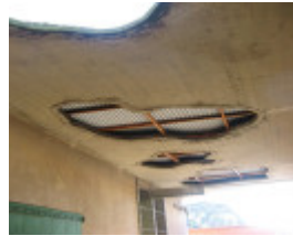
Maribyrnong substation cutouts in concrete roof
