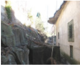
Maribyrnong substation quarry wall at rear
