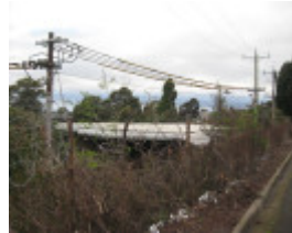
Maribyrnong substation view from above
