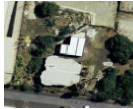
Maribyrnong substation aerial view
