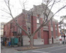
Carlton tram substation front and west side
