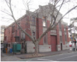
Carlton tram substation front and west side
