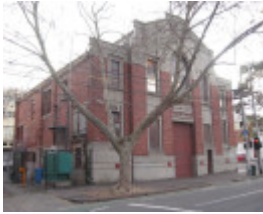
Carlton tram substation front and west side
