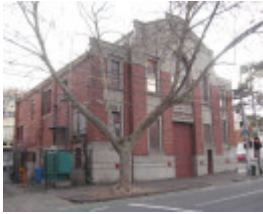
Carlton tram substation front and west side
