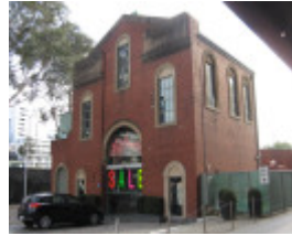
South Yarra tram substation
