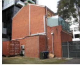
South Yarra tram substation rear view
