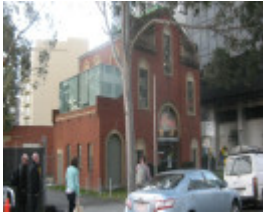
Tram substation Sth Yarra 5 Sep 2012 KJ (1).JPG
