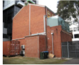
South Yarra tram substation rear view
