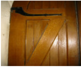
St Andrews Kirk Door Detail 01 Oct 03
