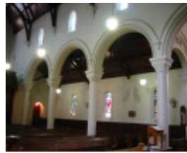
St Andrews Kirk Interior 04 Oct 03
