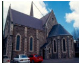
h00044 st andrews kirk ballarat north elevation oct03
