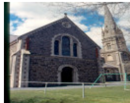
h00044 st andrews kirk ballarat west transept oct03
