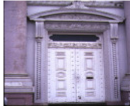
former commercial bank of austrialia bendigo detail entrance
